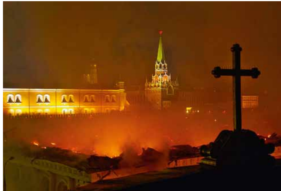
14.03.2004. A fire of the highest category of difficulty at the Moscow Manege
